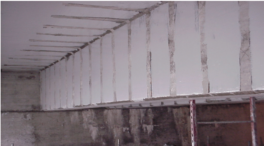
FIGURE 4. Installed laminate system.
