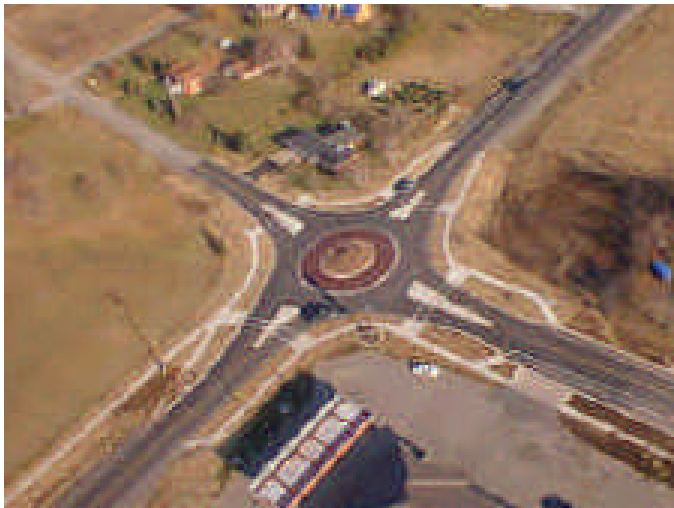
Figure 7-1. Lineville Road at Cardinal Lane
