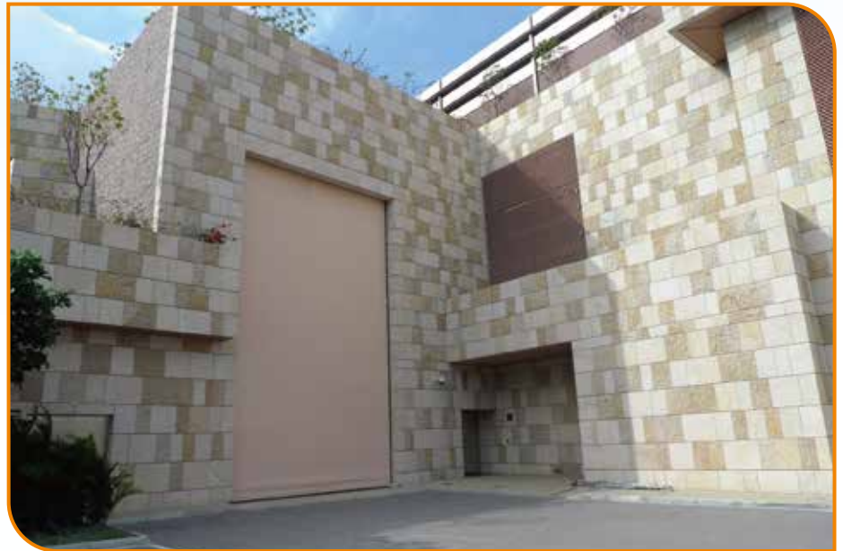
▲ Secure hangar storage facility. 保密飛機庫儲存設施。
