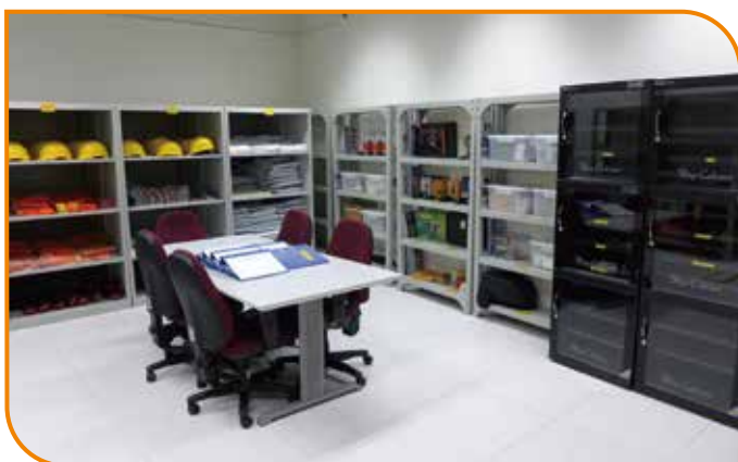
▲ Investigation Equipment Room. 調查設備室。
