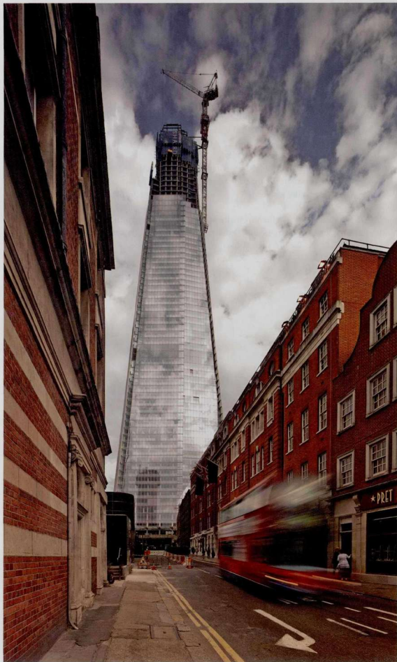
5 建造中外观/External view under construction (摄影/Photo, Nic Lehoucq)
