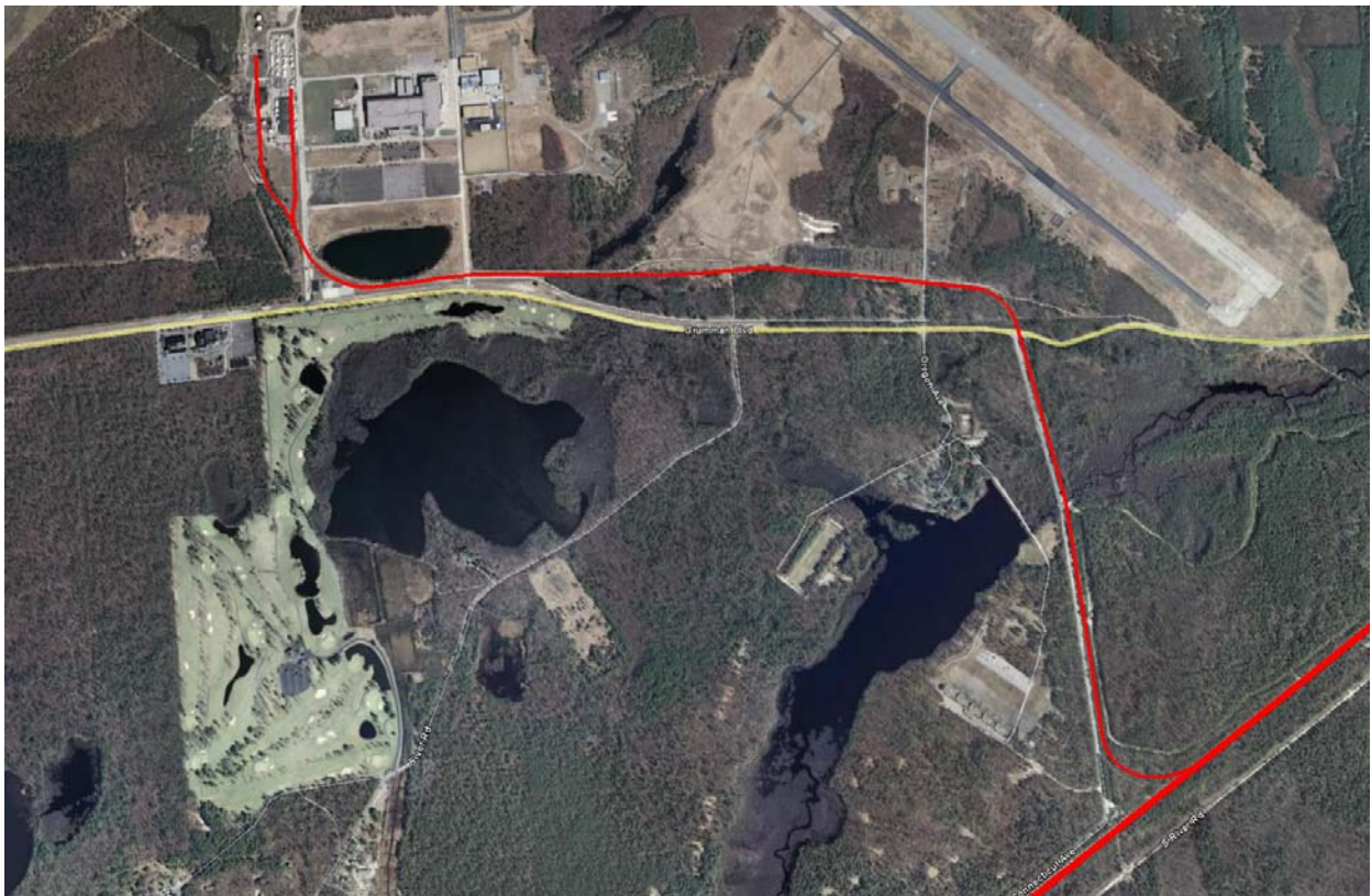
Rail Spur off of LIRR Mainline into Calverton Enterprise Industrial Park
