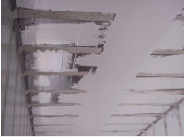
Figure 4A. Primer and putty applied at marked locations.
