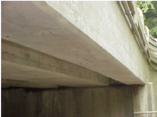
Figure 4B. Installed FRP-laminate system in place (painted to match concrete color).
