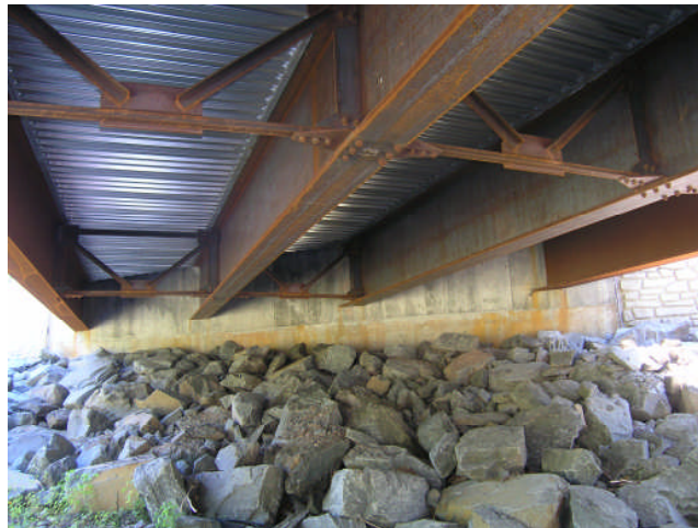
Figure 2: Example of a constructed FIAB
