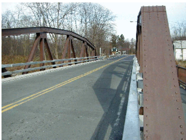
Figure 6. Bentley Creek bridge after rehabilitation.
