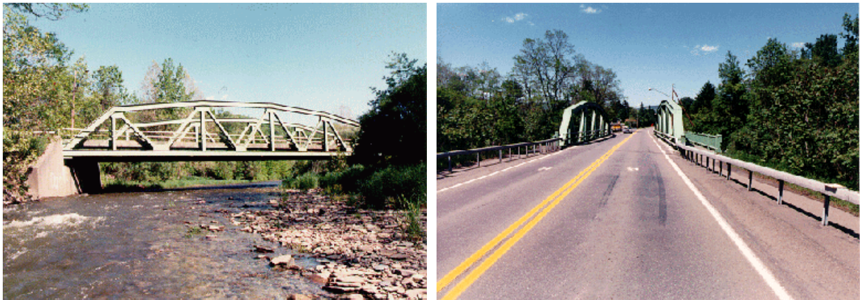
Figure 1. Views of Bentley Creek Bridge before rehabilitation.
