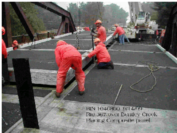
Figure 5. Composite deck panels being positioned with a crane.
