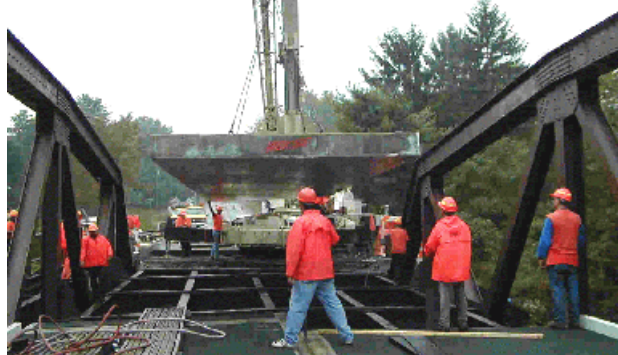
Figure 5. Composite deck panels being positioned with a crane.
