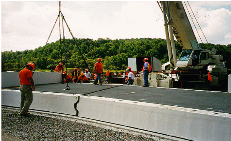
Figure 2. FRP superstructure's longitudinal shear-key.
