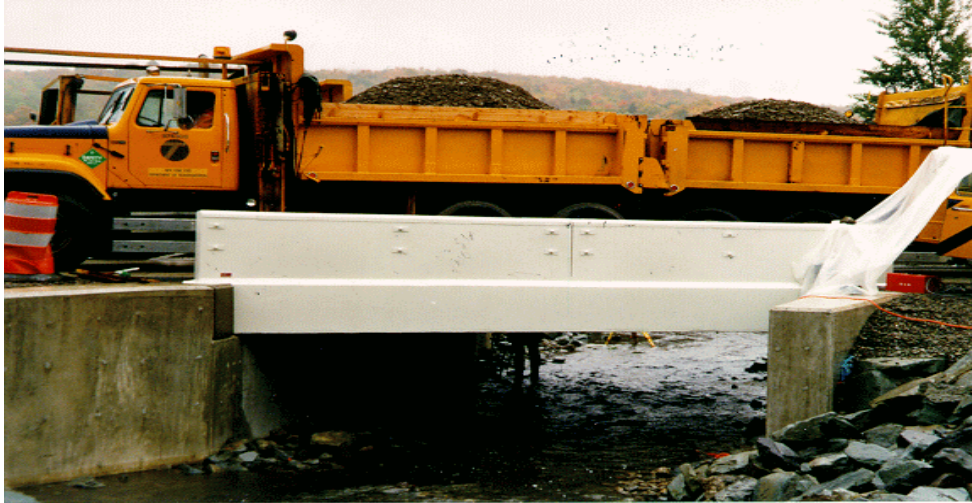
Figure 5. Proof-testing of the FRP Superstructure.
