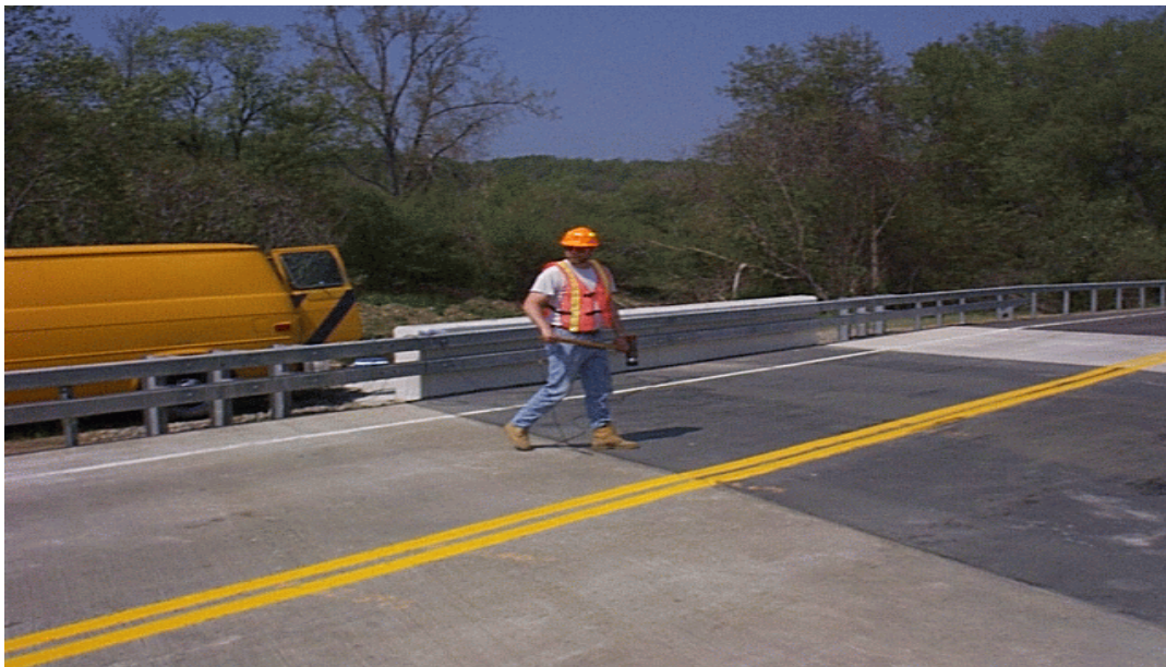
Figure 1. FRP superstructure.
