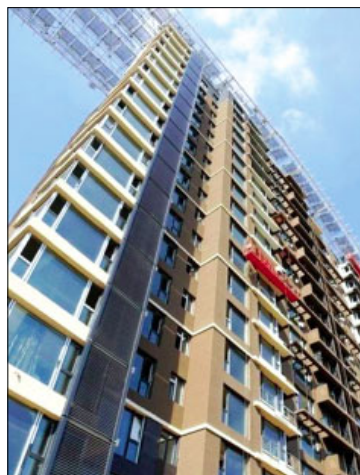
图6 可再生能源与建筑一体化 Fig.6 Integration between renewable energy source and building
