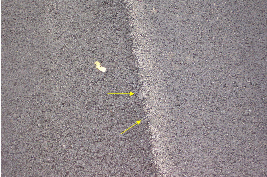
Photo 9: Adhesive Beads @ Surface After Rolling
