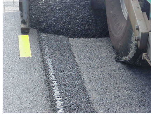
Photo 8: Paving Second Lane
