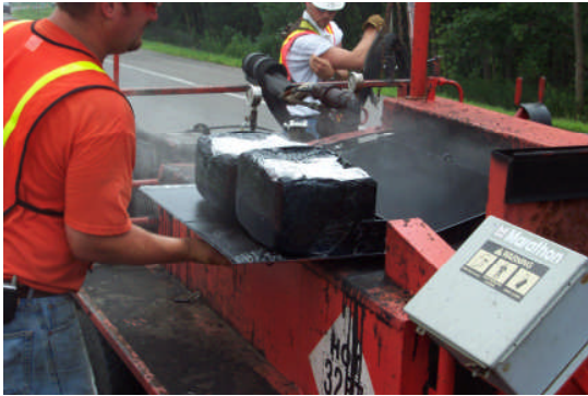
Photo 1: Loading Adhesive into Melting Pot
