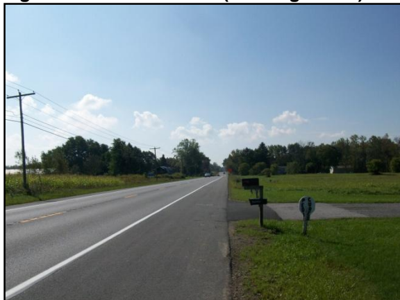
Figure 3 – NYS Route 77 (Looking South)
