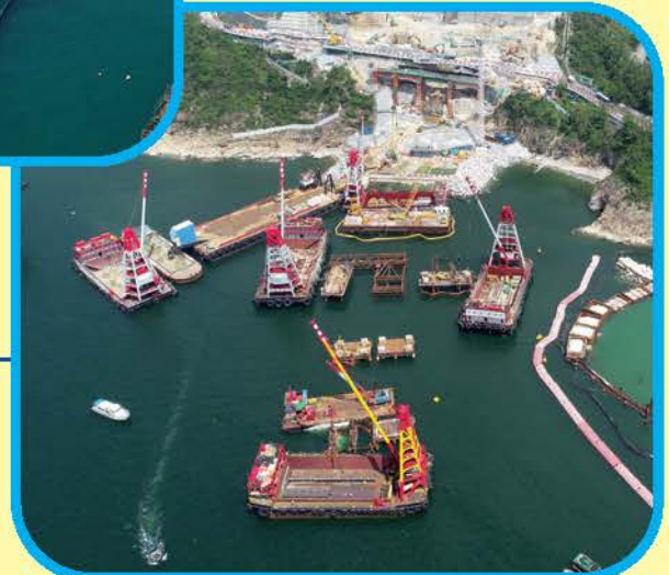
海上勘探及樁柱工程 Marine pre-drilling and bored piling works
