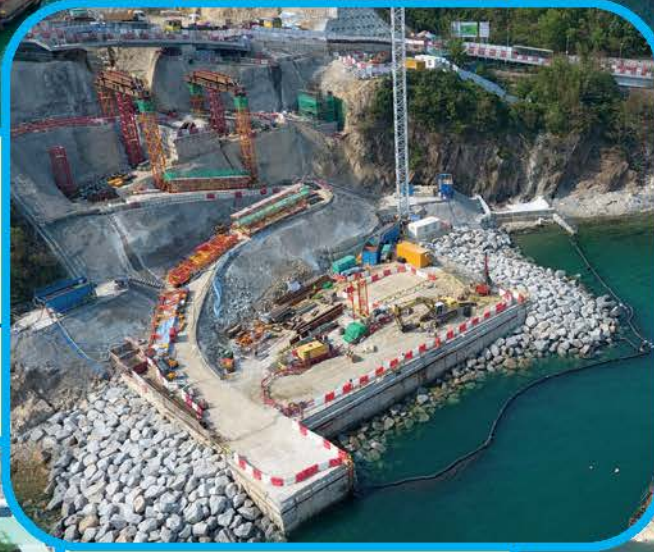
臨時躉船轉運站 Temporary barging point
