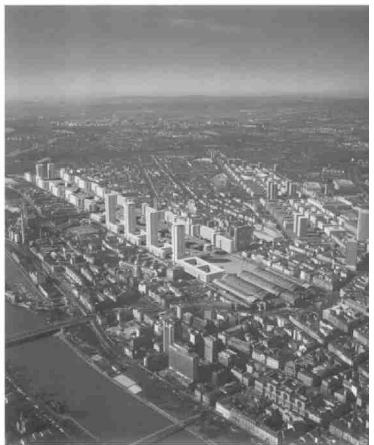
Urban Planning and Main Station, "Frankfurt 21" Bottom: Development area, potential development with focus on the "trade fair boulevard".
